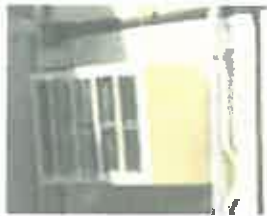
(2) 1-ton AC wall hung units stacked on left end access doors. Humistat: 60% humidity goal
